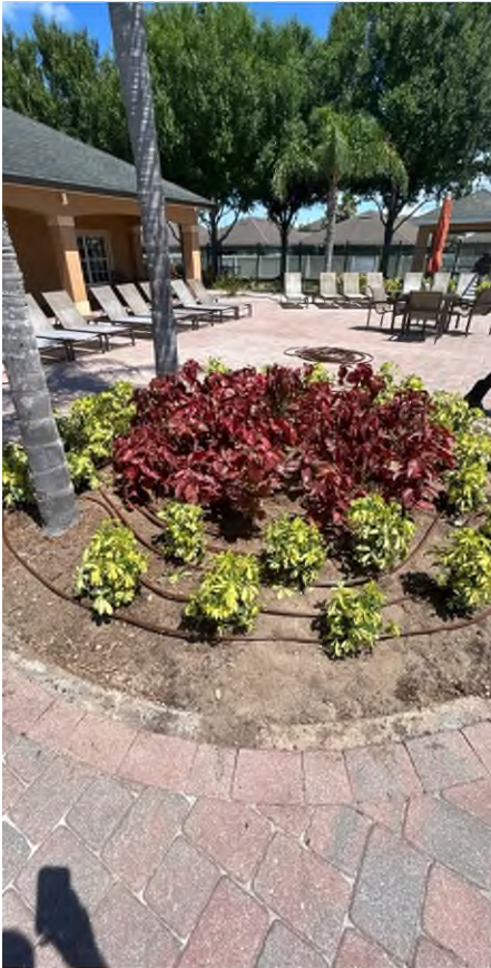
New drip in pool deck
