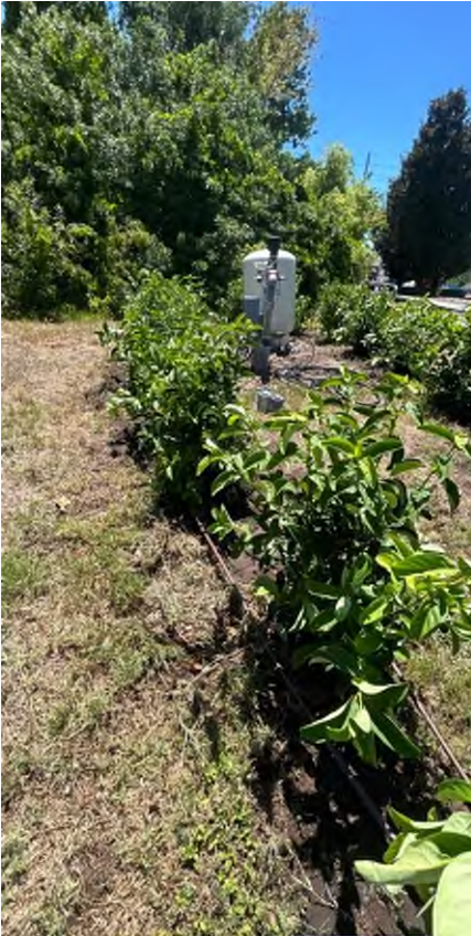
Drip below new plants around A-Controller and pump
